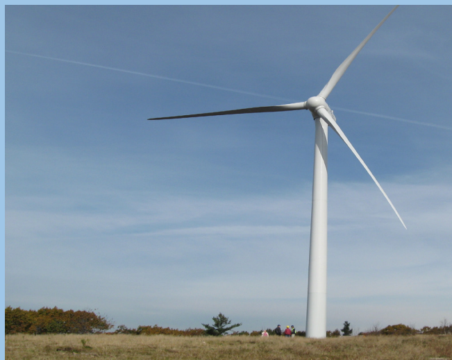
In 2009, the Princeton Municipal Light Department installed two 1.5 MW turbines. At that time, it was the largest wind power installation in Massachusetts. Photo: Sam Feinsilver.
