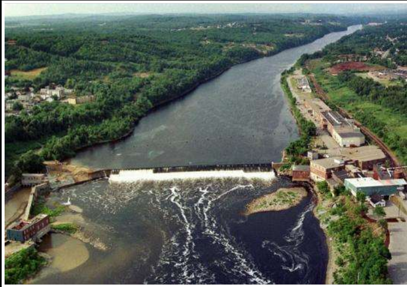
Edwards Dam, Kennebec River, built 1837 (Augusta, Maine) 3.5 MW!
