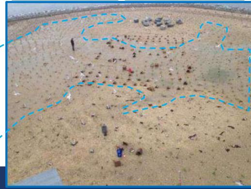
Installed cobble drainage ditches, connected to cobble ring, which was connected to revetment at low points of island (\*)
